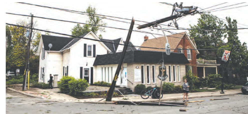
Hydro poles along Brock St. E. snapped in two. Photo by John Cavers
