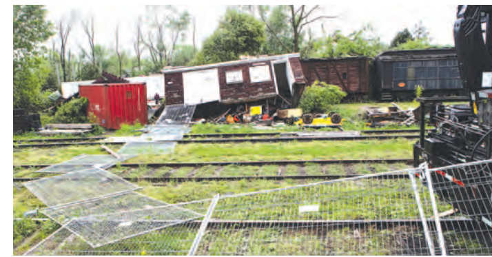
Devastation at the York-Durham Heritage Railway yard. Photo by John Cavers
